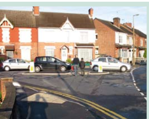
New pedestrian crossing facilities on all four arms at the busy Dallow Street / Victoria Crescent crossroads. This benefits three schools and the local community.
