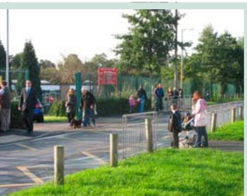
Pedestrian guard railing to segregate children from vehicles at Belvedere Junior School.
